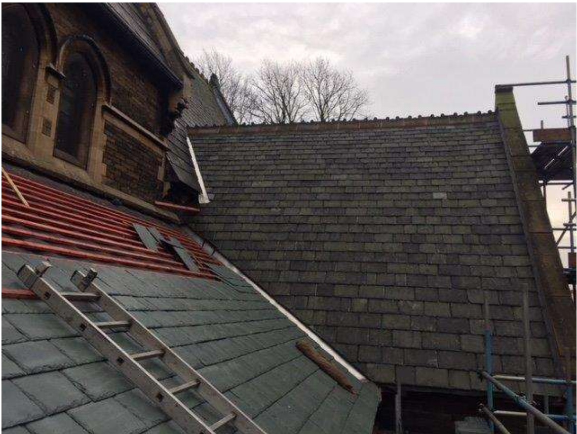
VIEW LOOKING EAST TO COMPLETED SOUTH TRANSEPT WEST SLOPE
