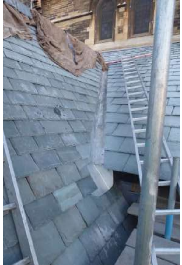
SOUTH PORCH/SOUTH AISLE VALLEY
