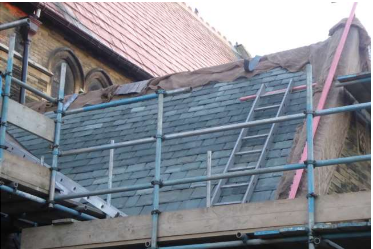
SOUTH PORCH, WEST SLOPE – RIDGES PROTECTED AFTER RE-LAYING
