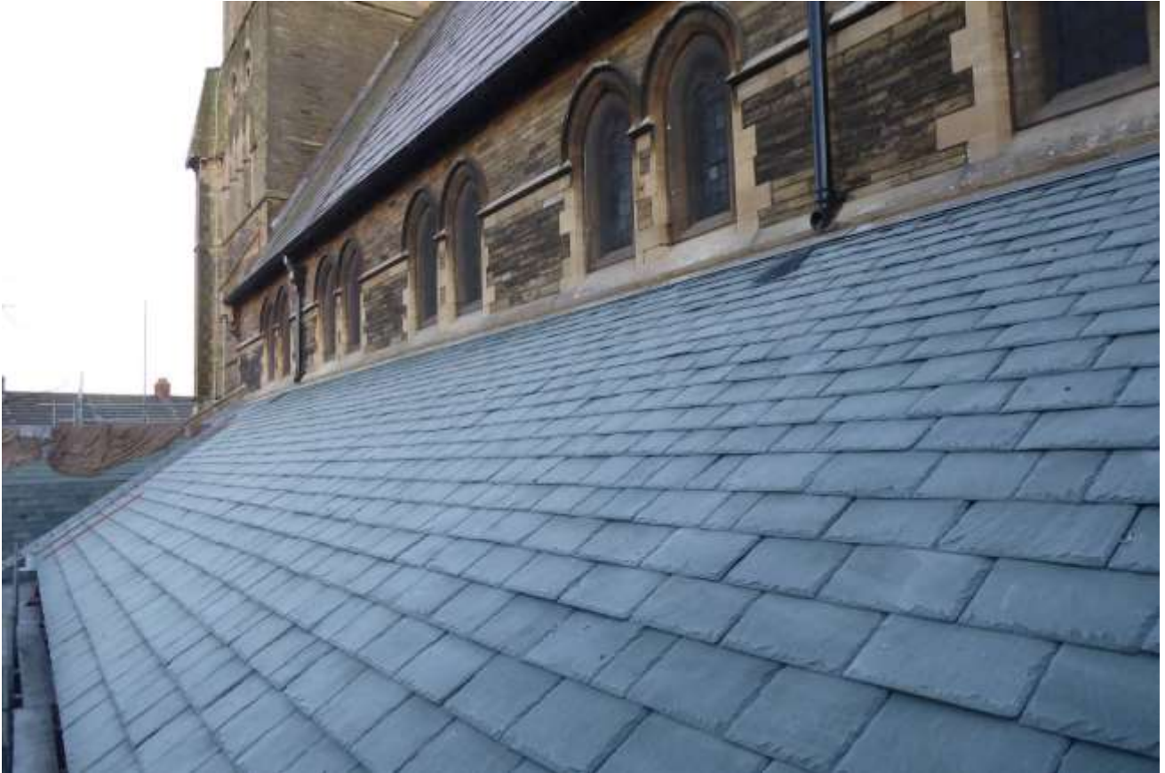
VIEW LOOKING WEST ALONG COMPLETED SOUTH AISLE ROOF
