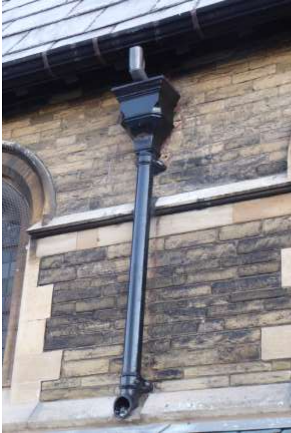
NEW CLERESTOREY DOWNPIPES
