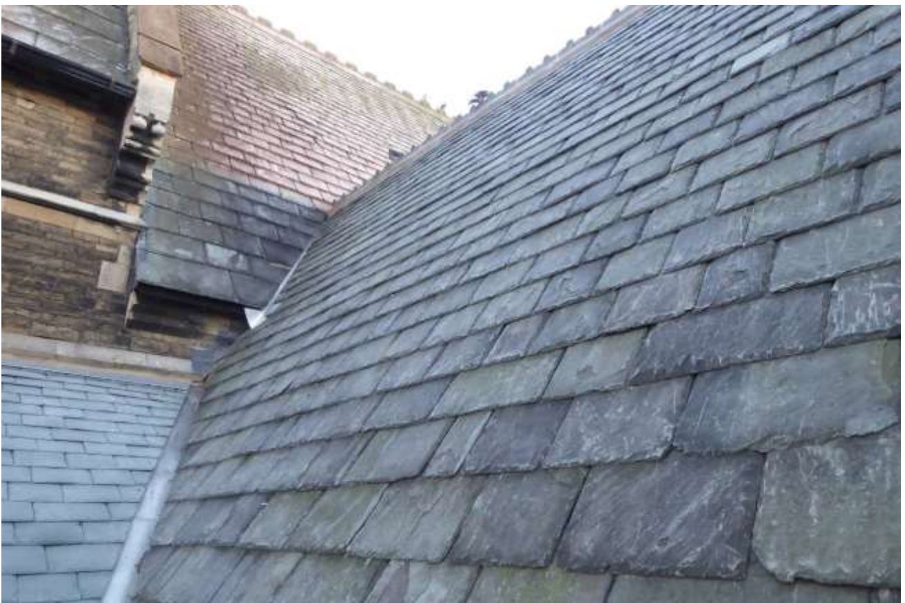
VIEW LOOKING NORTH ALONG COMPLETED SOUTH TRANSEPT SOUTH SLOPE
